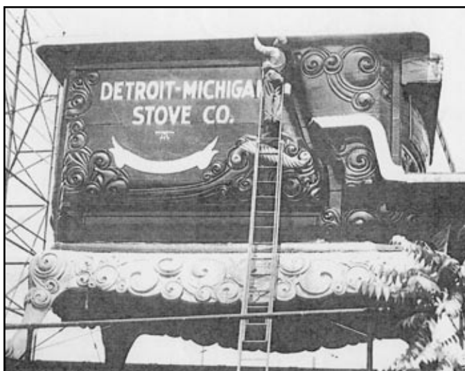
Painting the mammoth structure in the 1920s
